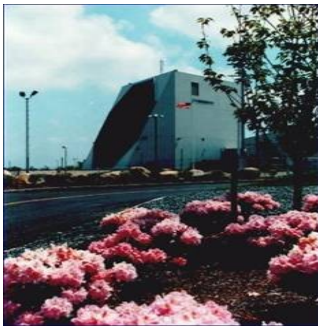
This photo from the internet shows the installation at Beale AFB. It looks like a giant speaker about 20 stories tall!
